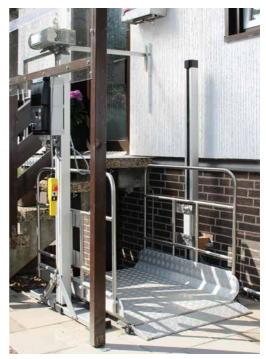
In addition to the dead man's operation and the soft start mechanism, the control unit has a lot of other functions. It is possible to set the speed parameters and the acceleration ramp.
