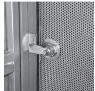
panel firmly bolted together
